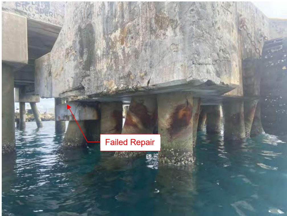
Photo 16 – Breasting Dolphin H
