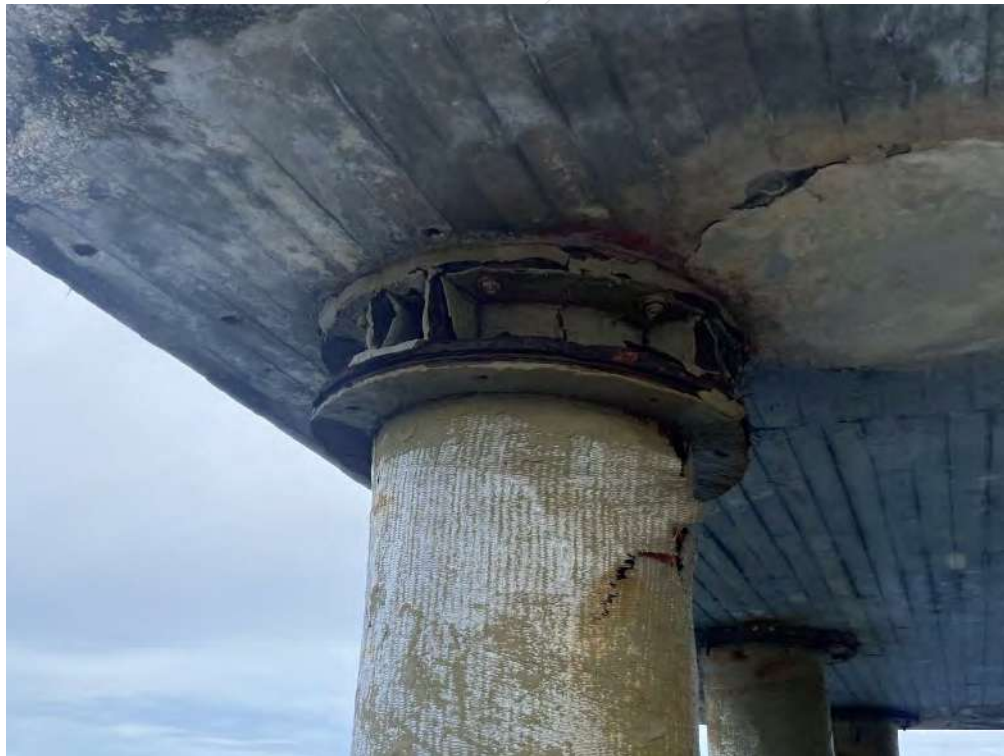
Photo 8 – Mooring Dolphin A
