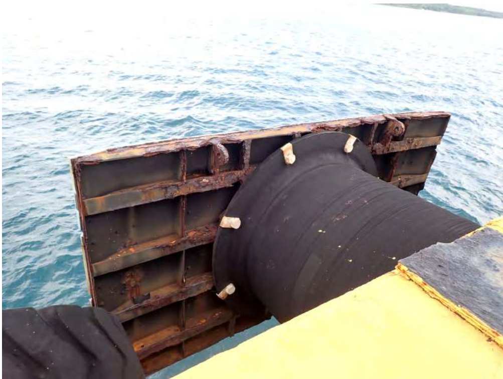
Photo 17 – Breasting Dolphin D
