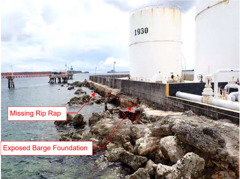
Photo 5 – Peninsula West of Trestle
