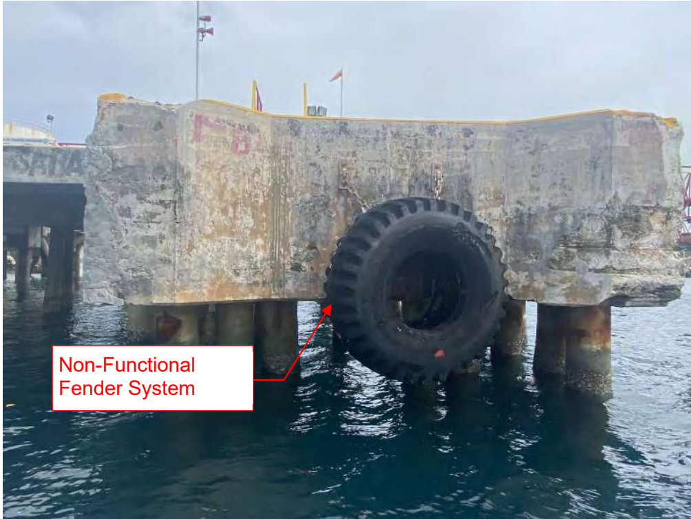
Photo 15 – Breasting Dolphin H
