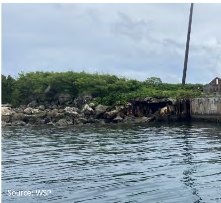
Photo 33: Hotel Wharf (Exposed Anchor Wall)
