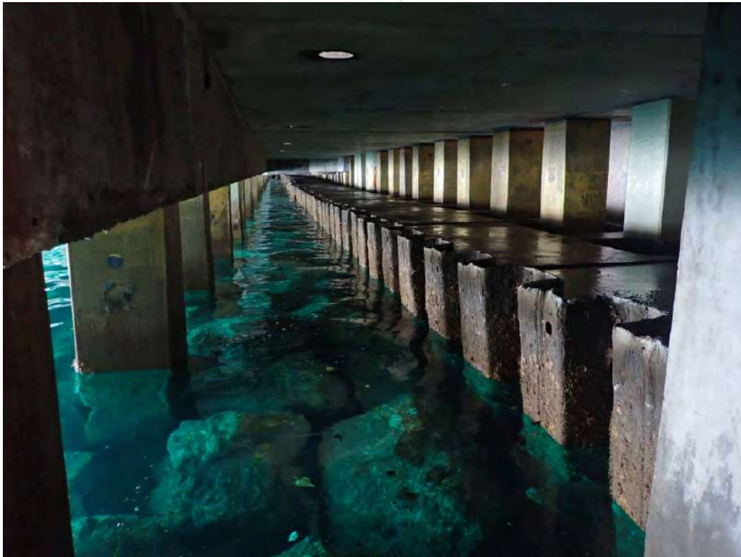
Photo 18 – Typical Landside Sheet Pile Wall
