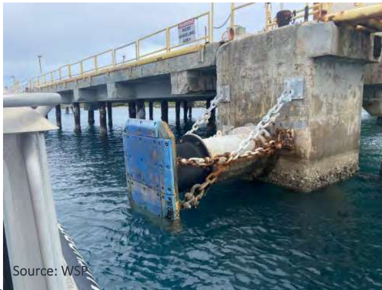
Photo 31: Golf Pier (Pier and Breasting Dolphin)
