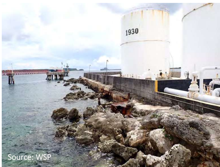
Photo 27: Peninsula West of Trestle (Exposed Barge Foundation)
