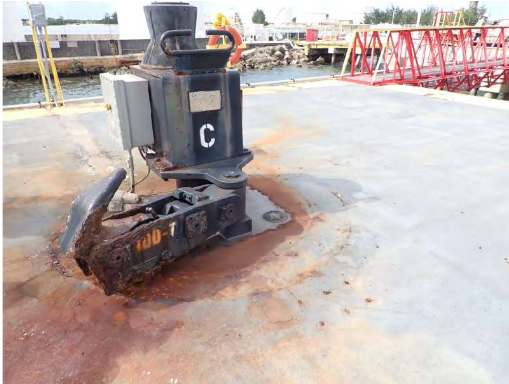
Photo 11 – Breasting Dolphin C
