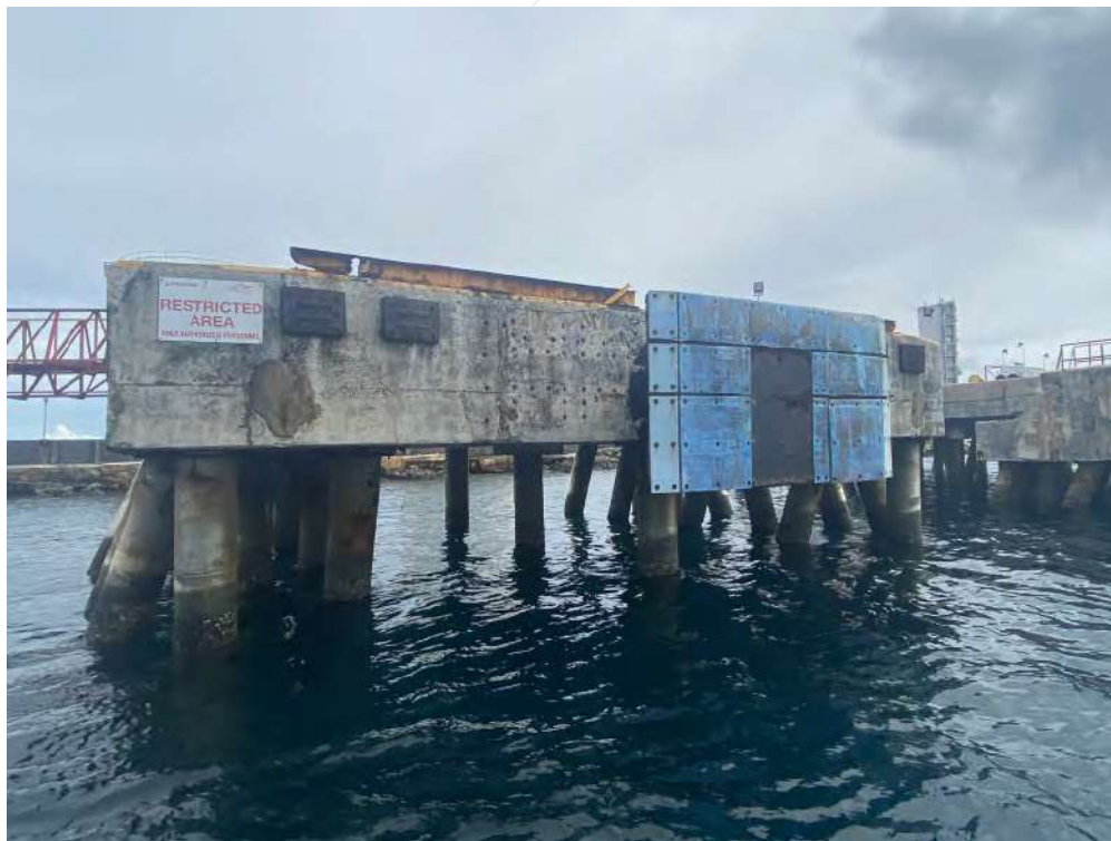
Photo 12 – Breasting Dolphin C
