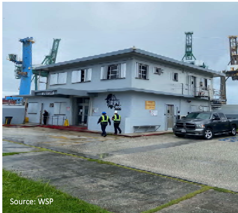
Photo 15: New Operations Building
