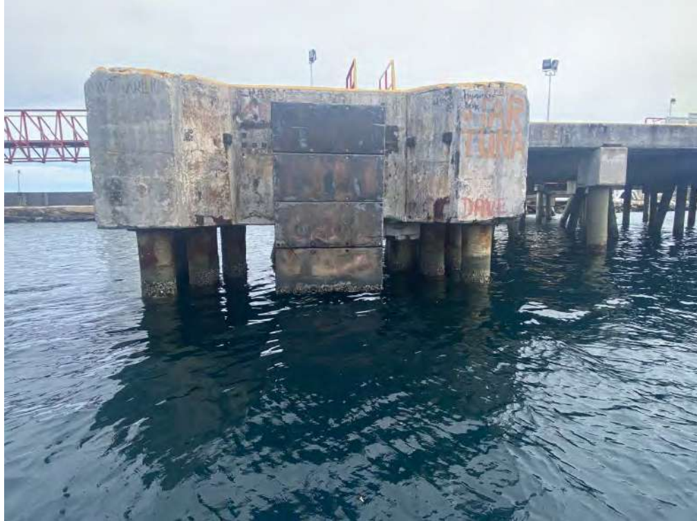
Photo 13 – Breasting Dolphin G
