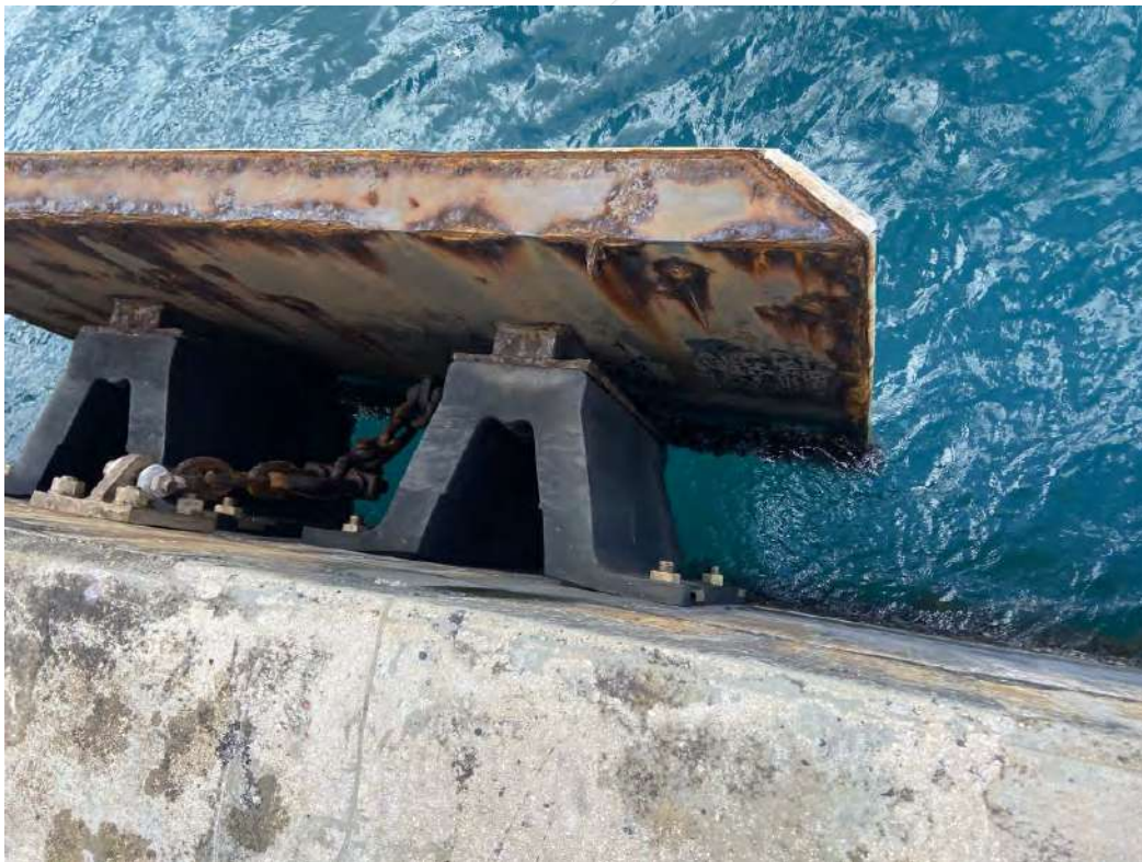
Photo 12 – Berth F4 Typical Fender Panel
