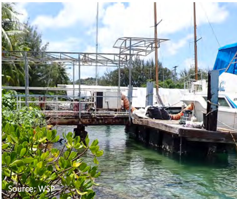
Photo 42: Harbor of Refuge (Long-Term Moorage Structure)
