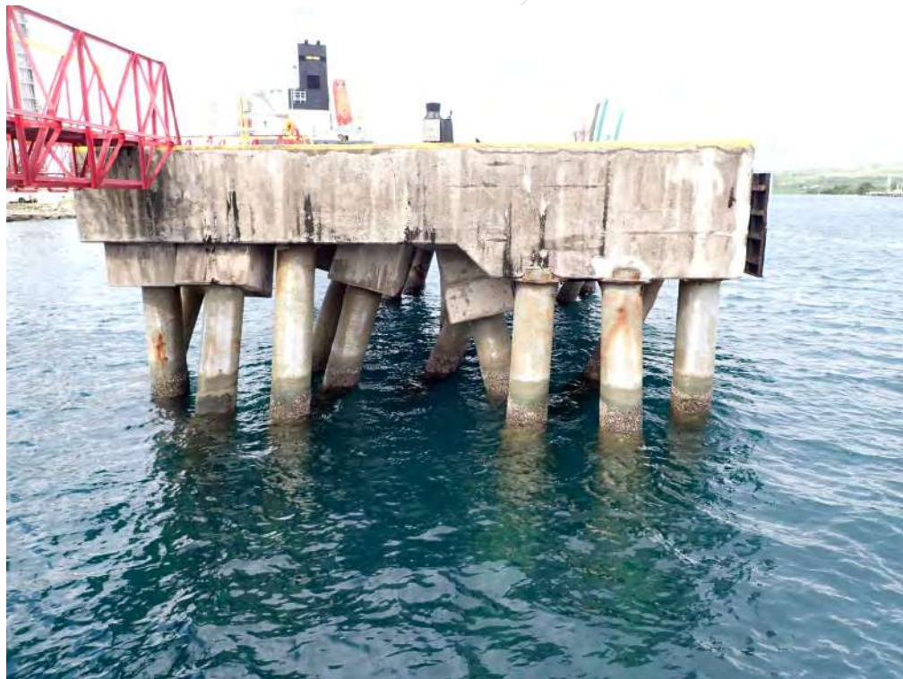
Photo 14 – Breasting Dolphin G
