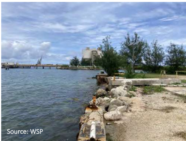
Photo 29: Seaplane Ramp Bulkhead
