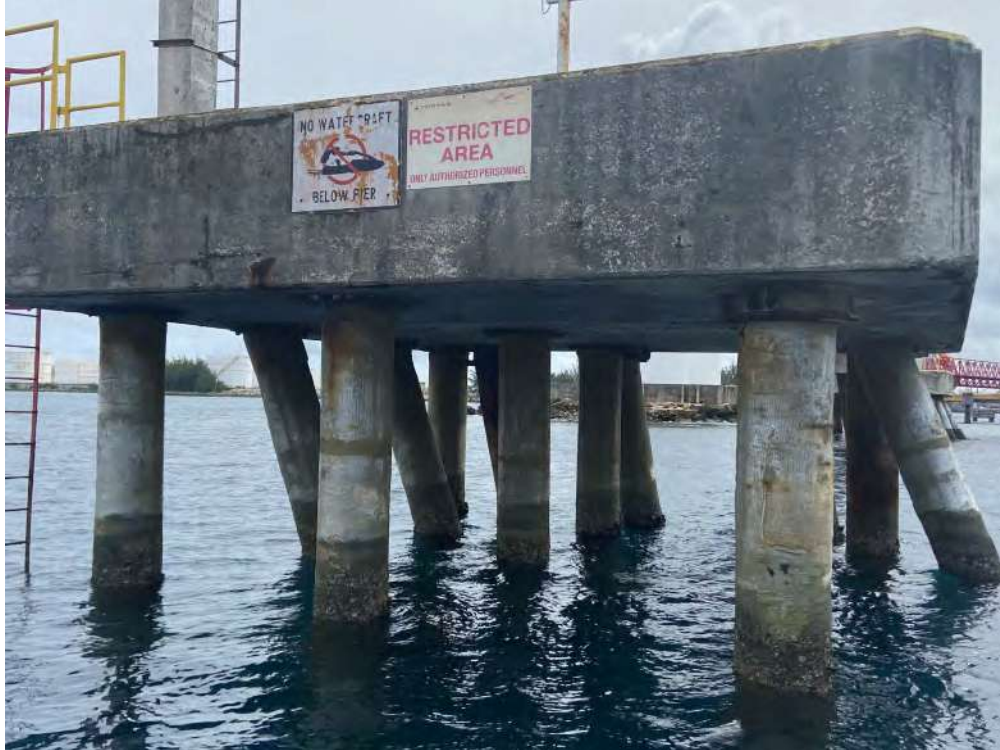
Photo 7 – Mooring Dolphin A
