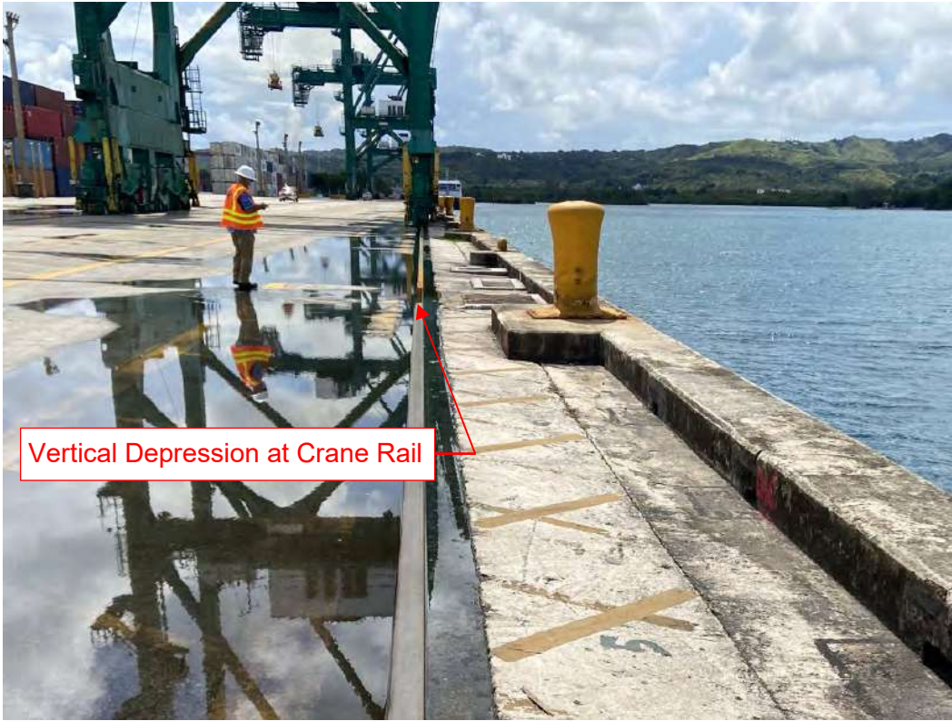
Photo 11 – Berth F4 Depression at Crane Rail
