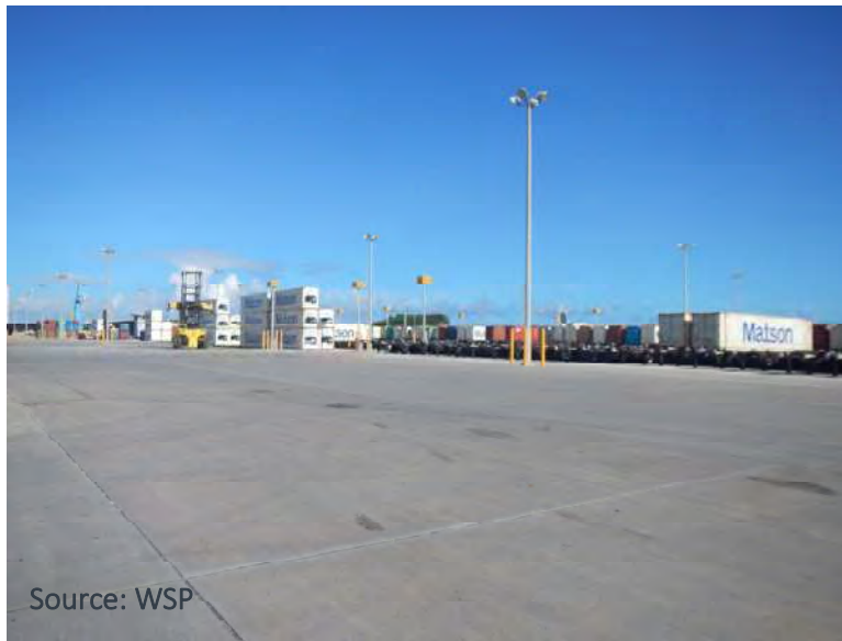
Photo 8: Container Yard Pavement
