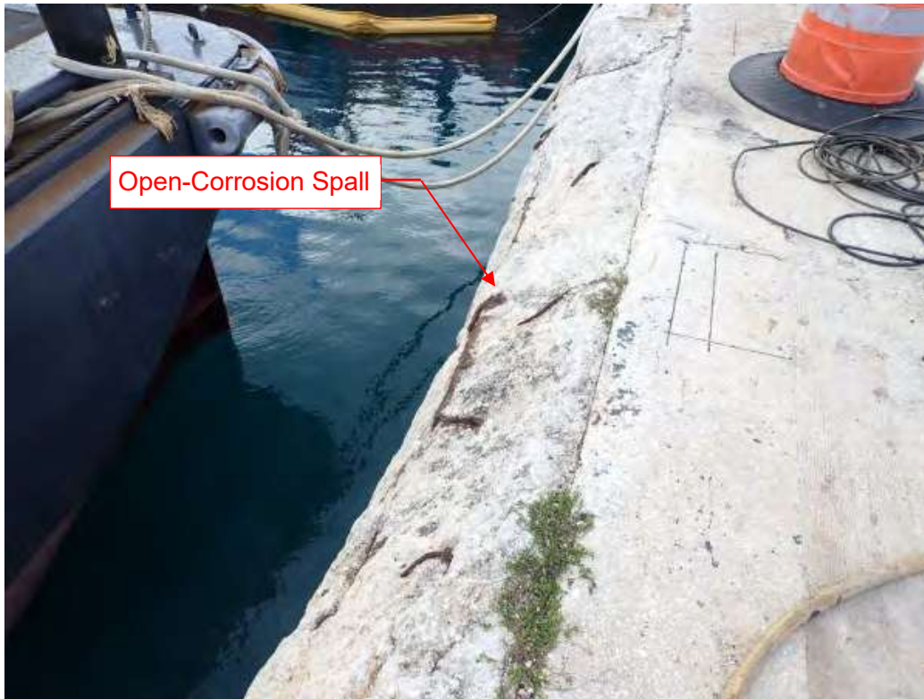
Photo 3 – Berth F2 Typical Concrete Pile Cap
