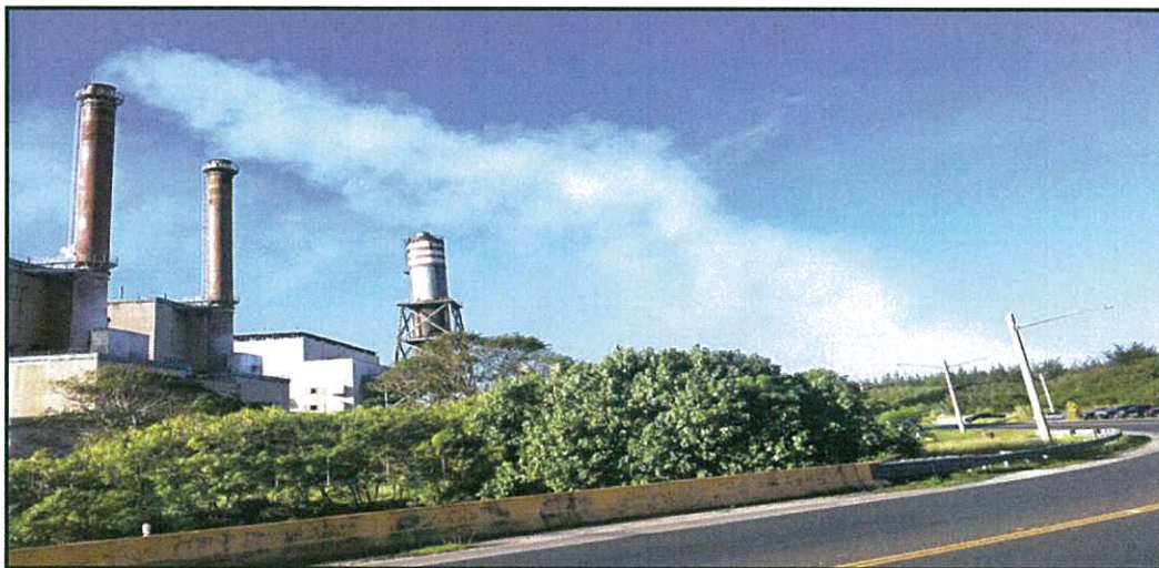
Guam Power Authority Cabras Nos. 1 and 2.
