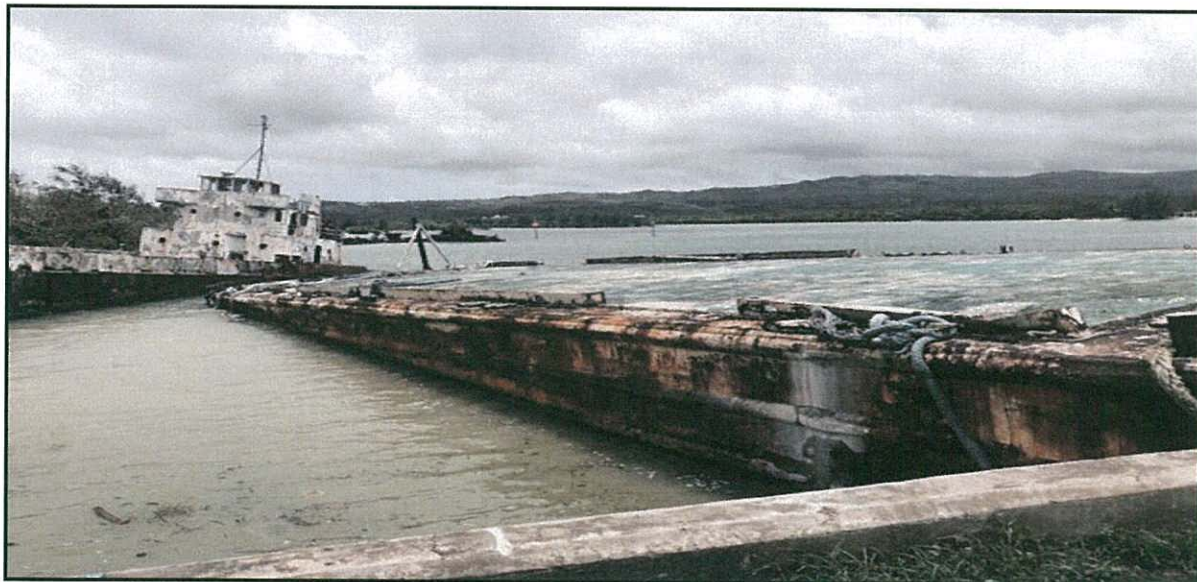
Barge broke loose at F6 and caused damaged to the wharf.
