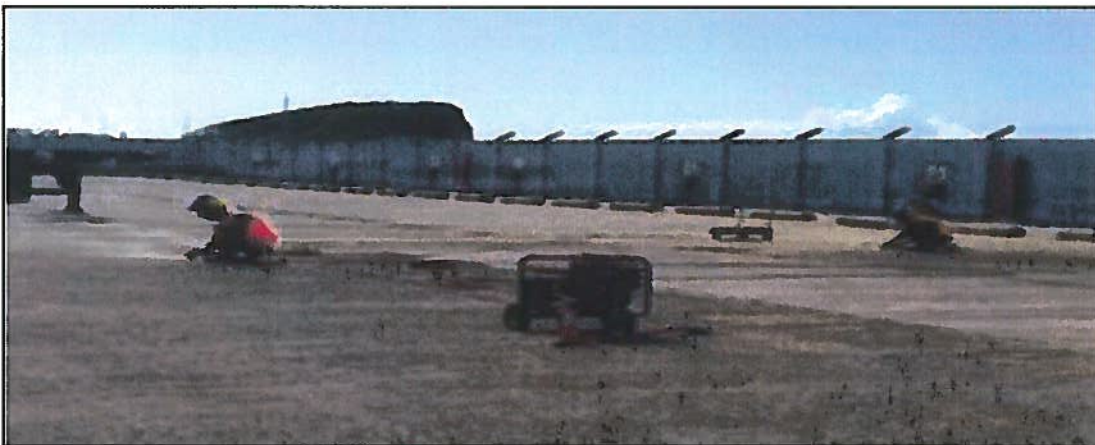
Port Contractor Canton Construction employees removing old striping in the Reefer Section of the yard.
