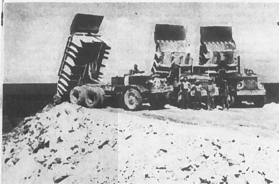
Fig. 7 Side dump equipment (at top) delivers heavy stone on the seaward face. Bulldozers supplement the dumping where necessary. Below: The fill is advanced by trucks that back up for end dumping.
