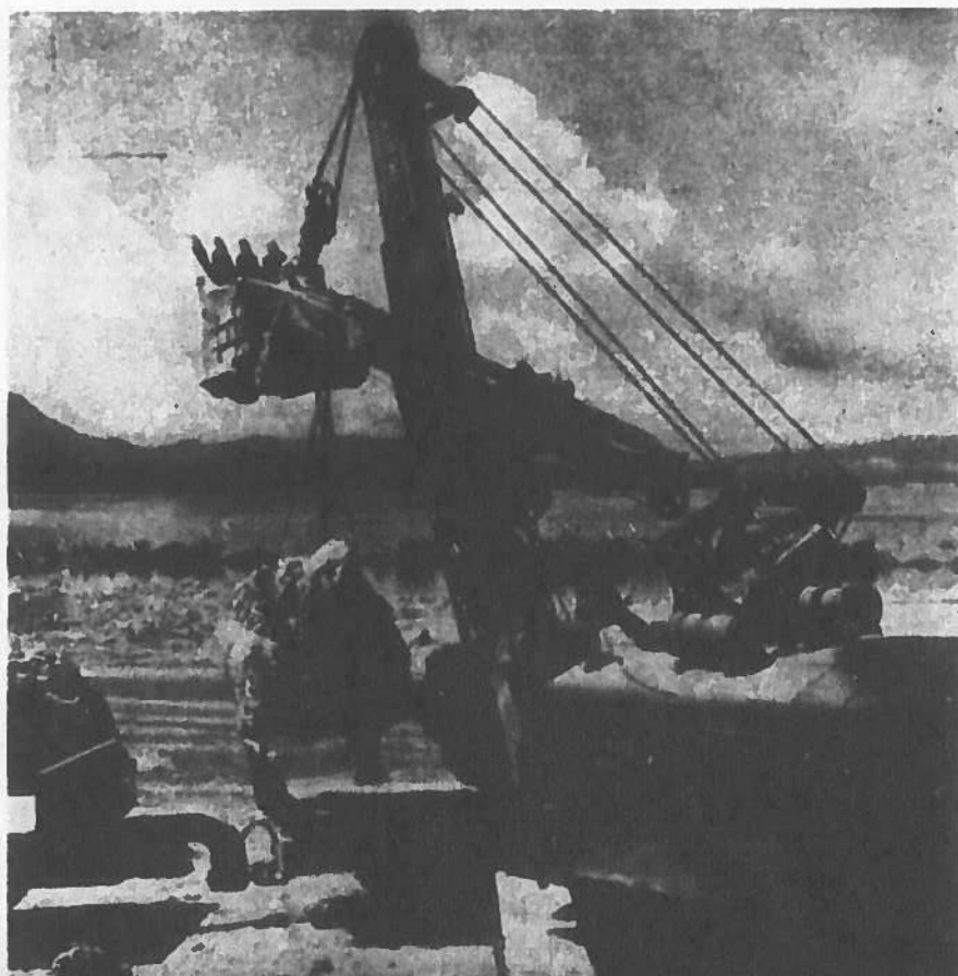
Fig. 4. Wire rope slings attached to dipper sticks enabled each shovel to handle rock of largest size as well as quarry run material.
