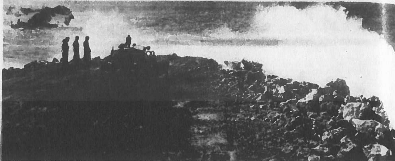
Fig. 1. The breakwater at this point is unprotected from the open sea. Concrete barges at left were wrecked by a typhoon.
