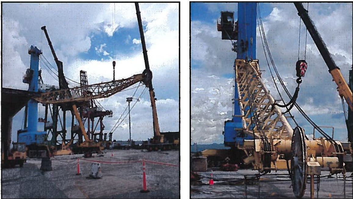
Smithbridge removes the boom from the Mobile Harbor Crane.
