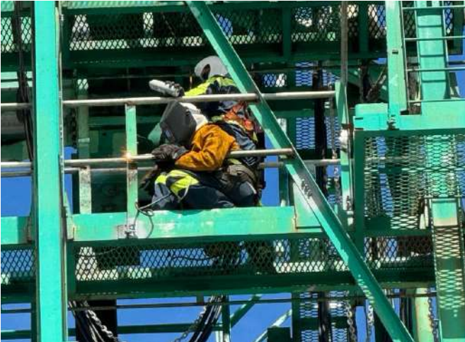
Equipment Maintenance crew perform routine upkeep on Gantry 4 on May 3, 2024.
