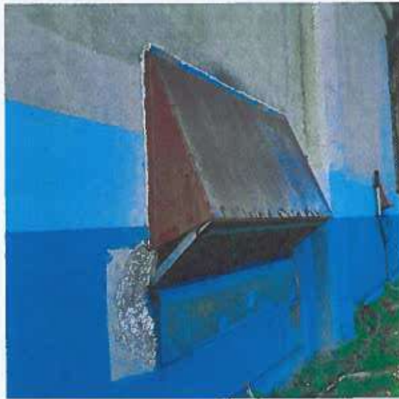
Figure 3: Exhaust Vent to be Removed and Replaced
