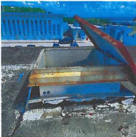
Figure 14: Roof Hatch to be Removed and Replaced
