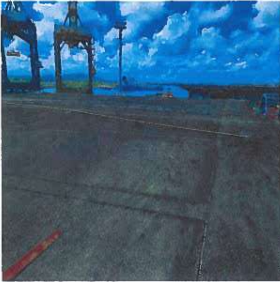
Figure 16: Welding Shop Roof Top
