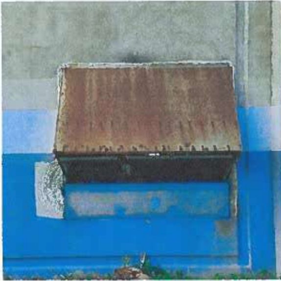
Figure 1: Exhaust Vent to be Removed and Replaced
