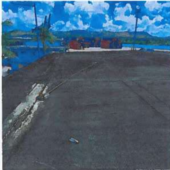
Figure 18: Welding Shop Roof Top
