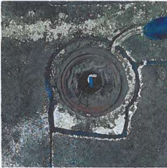
Figure 10: Roof Drain to be Removed and Replaced
