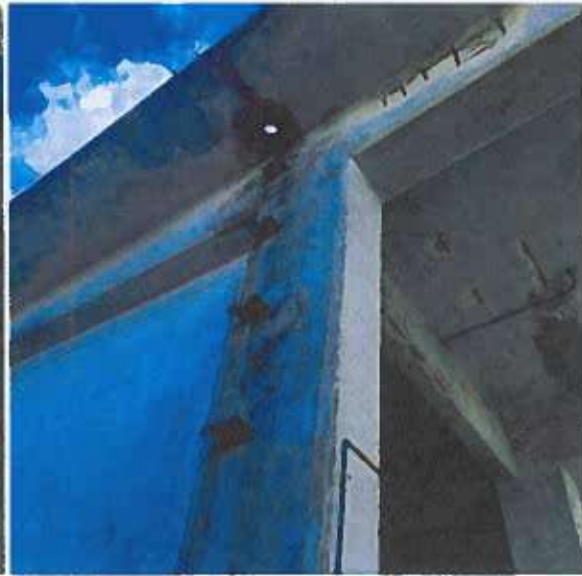
Figure 11: Downspout Location (West)
