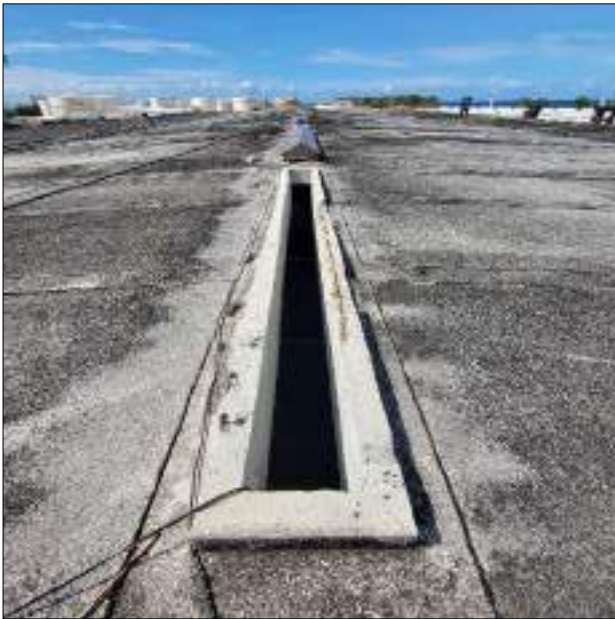
Figure 7: Bay 4 – Roof vent opening.
