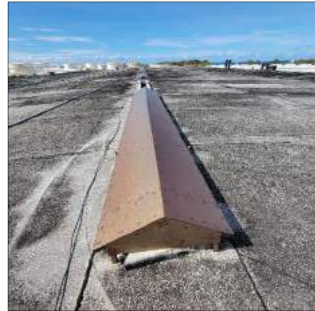
Figure 8: Bay 5 – Roof vent to be disposed.
