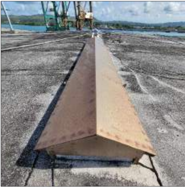
Figure 5: Bay 3 – Roof vent to remain.
