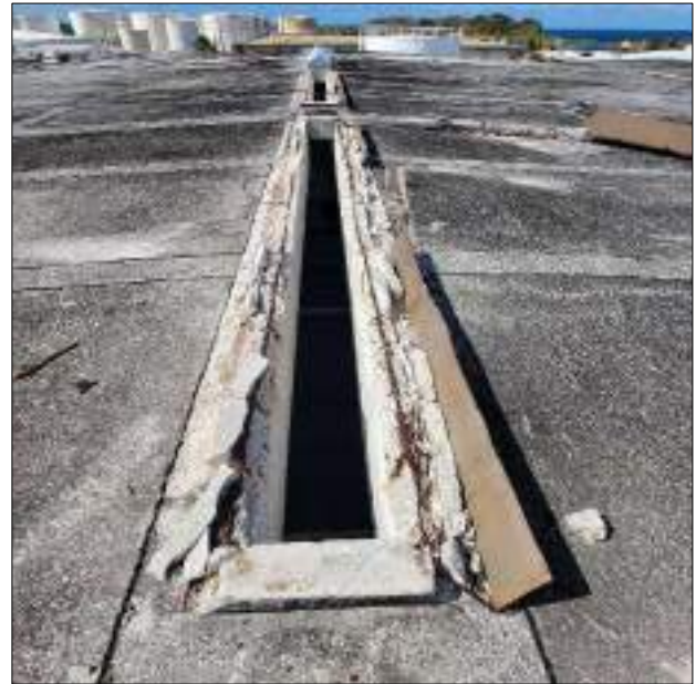
Figure 28: Bay 12 – Stainless steel sheets to be disposed.
