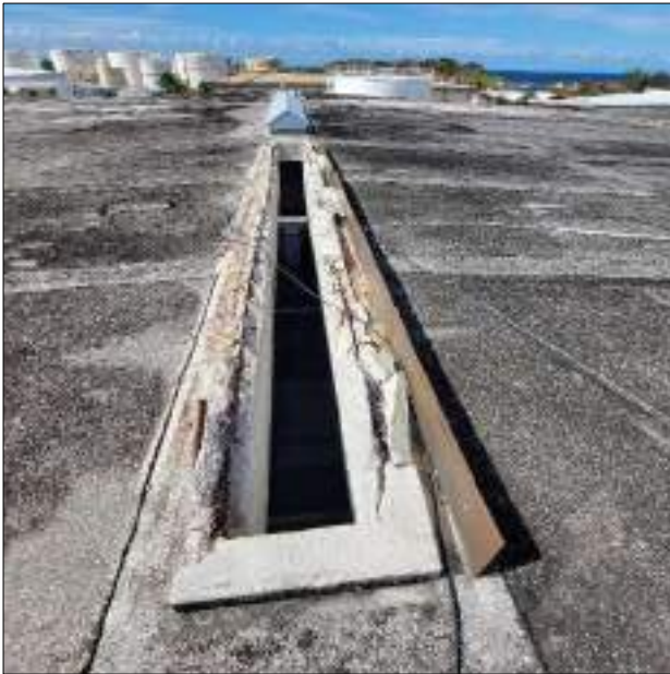
Figure 31: Bay 13 – Stainless steel sheets to be disposed
