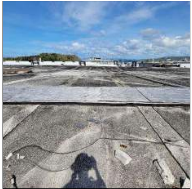
Figure 24: Bay 11 – Dispose of temporary cover.
