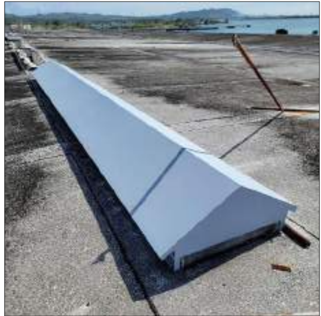
Figure 32: Bay 14 – Roof vent to remain.
