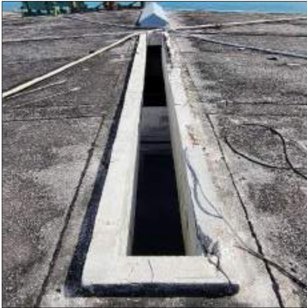
Figure 3: Bay 2 – Roof vent opening.
