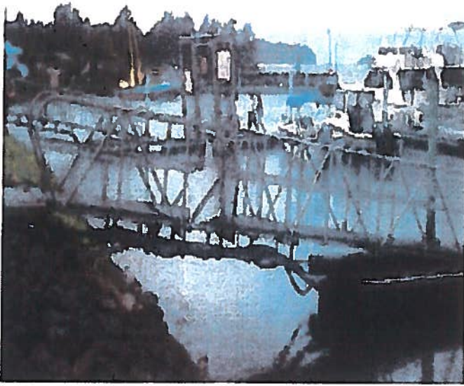
EXISTING GANG WAY ENTRANCE RAMP
