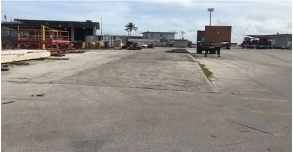
Figure 3: South Ramp of Devanning Area
