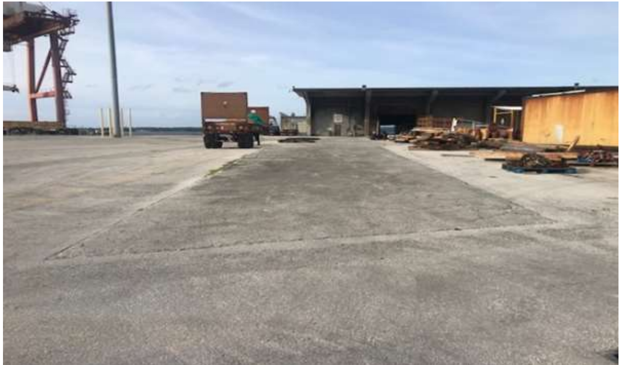
Figure 2: North Ramp of Devanning Area
