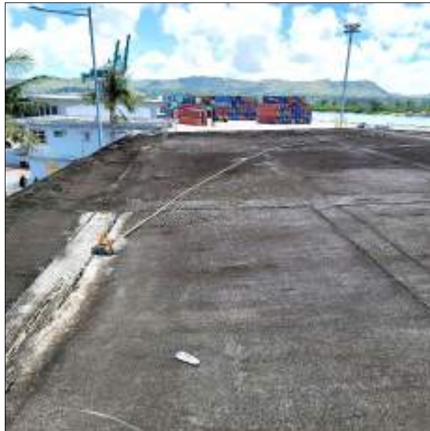
Figure 18: Welding Shop Roof Top
