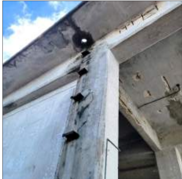
Figure 11: Downspout Location (West)
