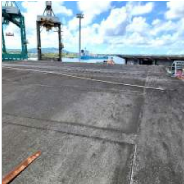
Figure 16: Welding Shop Roof Top
