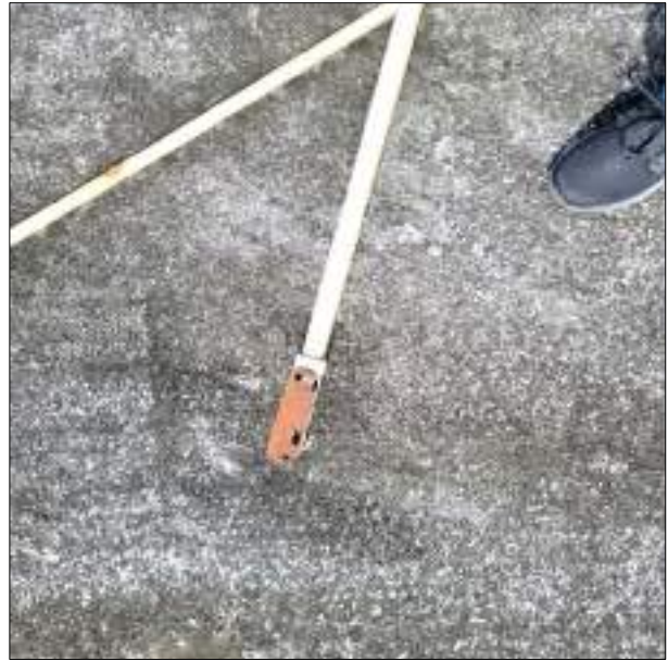
Figure 13: Electrical Line to be Removed and Relocated
