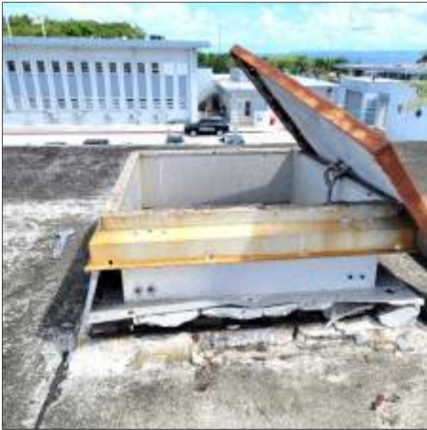
Figure 14: Roof Hatch to be Removed and Replaced
