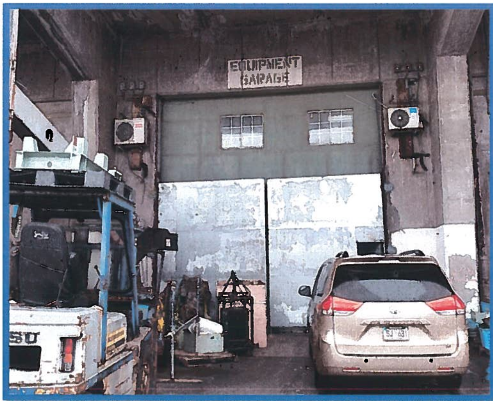
Bay 12 Landside: Tidewater Operations Roll-up Door 20'x20'
