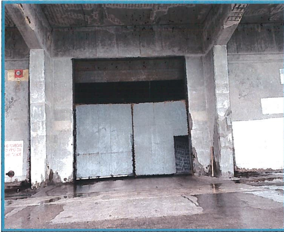
Bay 12 Waterfront side: Tidewater Operations Roll-up Door 20'x20'
